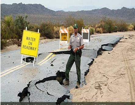
A flood damaged roadway in the southwestern U.S. (photo credit: NPS)
